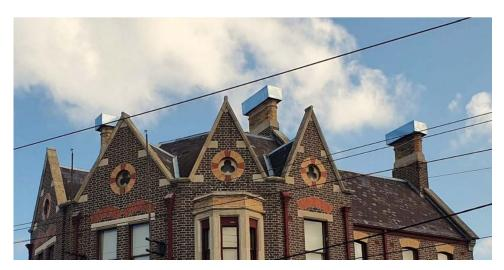
Above left: The front cover of the Conservation Management Plan (November 2022). Above right: The detailed image shows the temporary metal caps on the main chimneys, designed to protect the stone tops until repairs can be completed.
